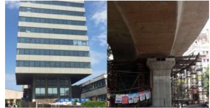
Fig. The Elephant with Horse's legs and the offset column [https://interestingengineering.com/21-engineering-and-design-failures]
